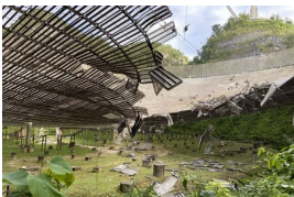
Arecibo Observatory's massive radio dish has a 30m gash in it UCF/Arecibo
